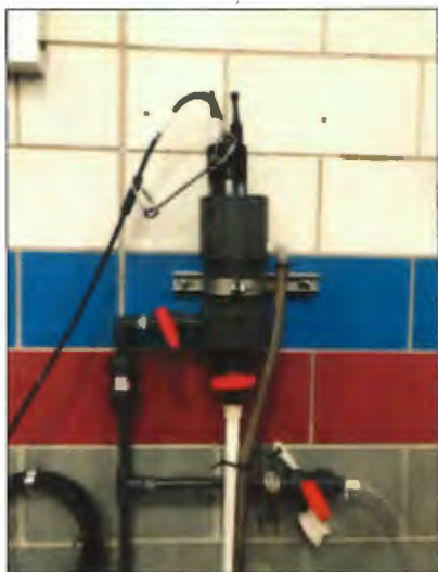
Installed multi-parameter Sonde probe monitors and reports changes in water quality parameters.
